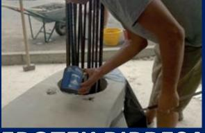
Two-component solvent-free epoxy resin with extremely low viscosity for construction joints and structural bondings
